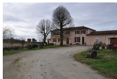
Logis principal. Phot. Caroline Bordes IVR72_20123300581NUCA
