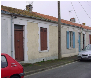
Façades. Phot. Yann Cussey IVR54_20071704322NUCA
