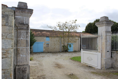
Le portail. Phot. Pierrick Barreau IVR54_20171709802NUCA
