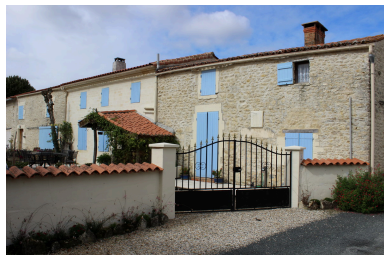
Le corps principal. Phot. Pierrick Barreau IVR54_20171709795NUCA
