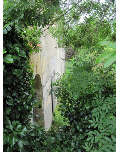
Elévation sud. Phot. Alain Beschi IVR72_20113302814NUC2A
