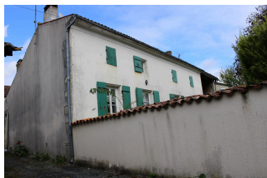
Le corps principal. Phot. Pierrick Barreau IVR54_20171709806NUCA
