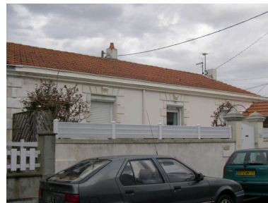
Façades. Phot. Christine Redien-Lairé IVR54_20061700532NUCA
