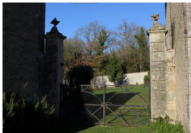
Le portail. Phot. Pierrick Barreau IVR54_20161710543NUCA
