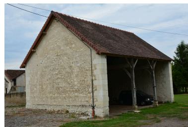
Hangar. Phot. Paul Maturi IVR75_20198604338NUCA
