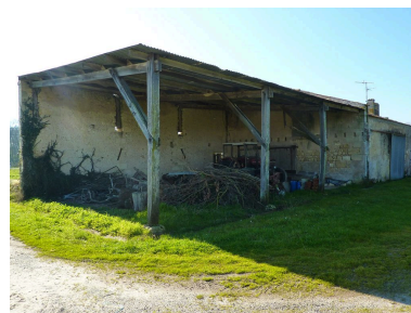
Hangar agricole. Phot. Jennifer Riberolle IVR72_20133300657NUC2A
